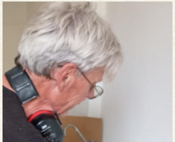
Installed the kitchen in the apartment
