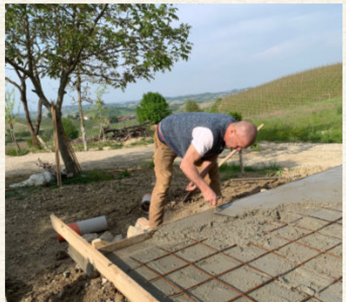
We already started the construction by laying the foundation
