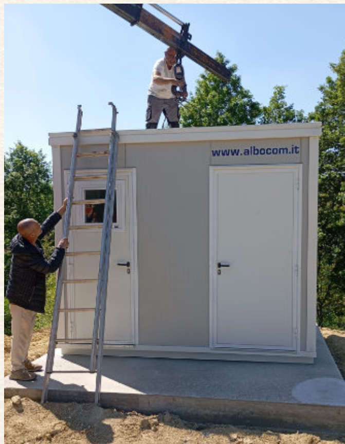
Installing the unit
